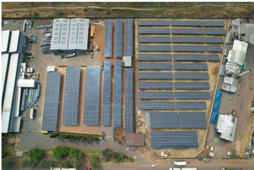
Maxion Wheels have installed a 2.9 MWp solar project to power the manufacturing plant. The panels cover a total area of 13 250m 2 , which is made up of an unused open area of 1 250m 2 , another ground mount open area of 9 500m 2 (2 000kWp) and the roof structures of the carpark account for 2 500m 2 (475kWp). The 1.6MWp Phase 2 of the project will be installed on the rooftop of the manufacturing facility
